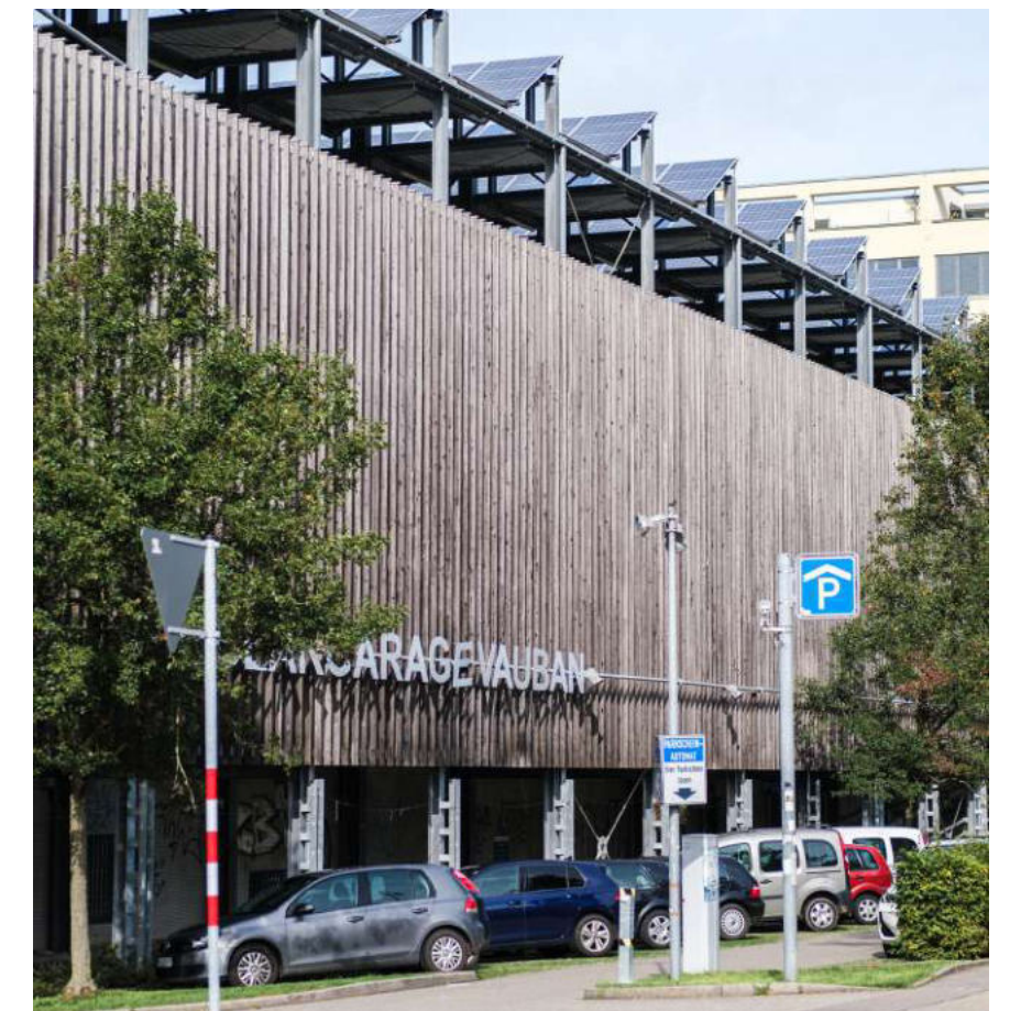
19 Quartiersparkhaus Vauban, Freiburg © Phillip Böhme
