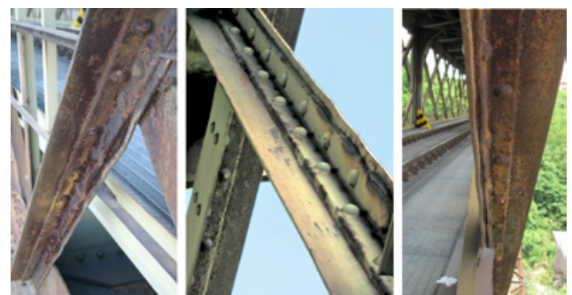
fig.4: Examples of members damaged by the corrosion (© Saisi and Gentile)
