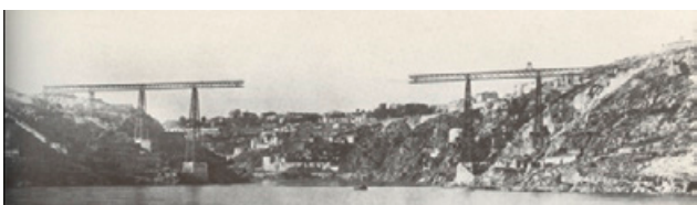
fig. 7: MARIA PIA BRIDGE - Abutments ready for arch construction to start by 19th Century photographs of unknown authors
