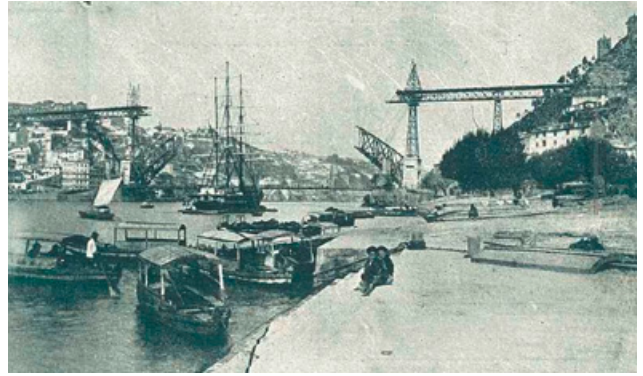
fig. 12: LUIZ I BRIDGE – arch initiating construction by 19th Century photographs of unknown authors
