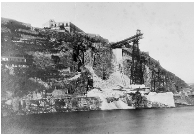
fig. 6: MARIA PIA BRIDGE - Column and deck on the right margin, advancing as cantilevers by 19th Century photographs of unknown authors
