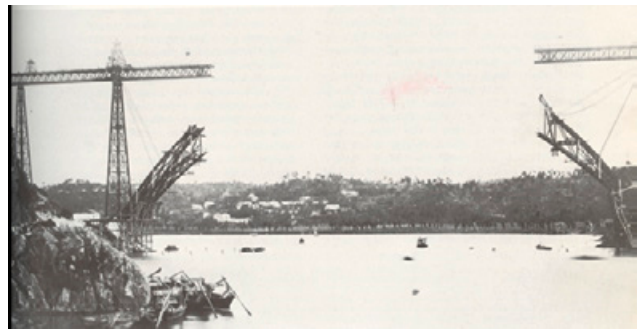
fig. 8: MARIA PIA BRIDGE – Arch construction with stays from top of columns by 19th Century photographs of unknown authors
