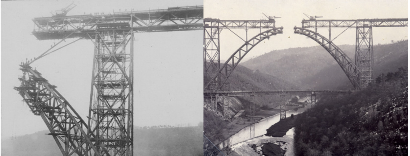
fig. 3: Müngsten Bridge under construction and short before completion of the steel truss arch in 1897 (© Stadtarchiv Solingen, MAN Museum und Historisches Archiv)
