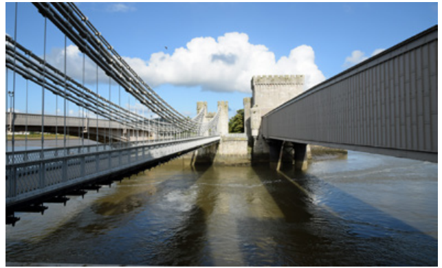
fig. 8: Telford's Conwy Suspension Bridge (1818) on the left, Stephenson's Conwy Tubular Bridge (1848) on the right (© Rolf Höhmann)
