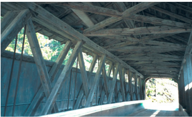
fig. 8: Howe girder system, Graubünden, Switzerland (© Pahl, Burkhard IGB, University of Leipzig)
