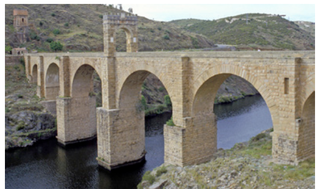
fig. 4: The Alcantara Bridge (ca. 105 AC) in western Spain shows the classic outlines of a roman arch bridge (© Rolf Höhmann)
